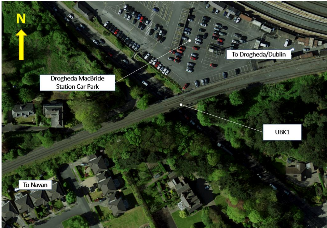
Figure 2-12: Aerial view of UBK1 (Source: OSI Aerial Mapping)
