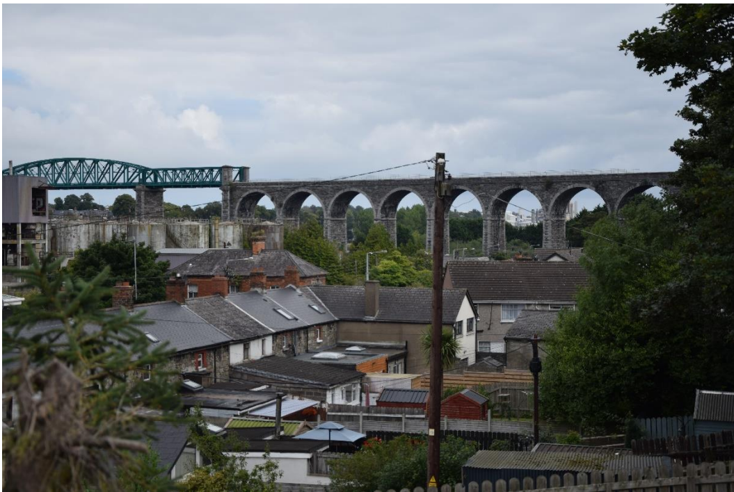
Figure 2-11: UBB82 Boyne Viaduct (Protected Structure LCC RPS DB-176)
